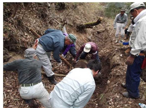
Small village support squad participating in waterway restoration activities
