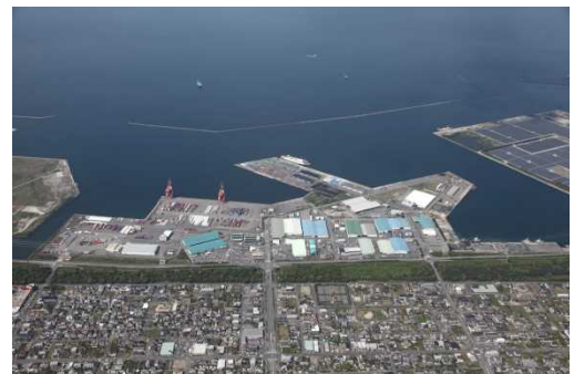
Distribution Base – Oita Port Ozai Region
